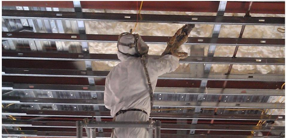
Following the installation of the spray foam, the team finished the process by using No Burn XD ignition barrier.
