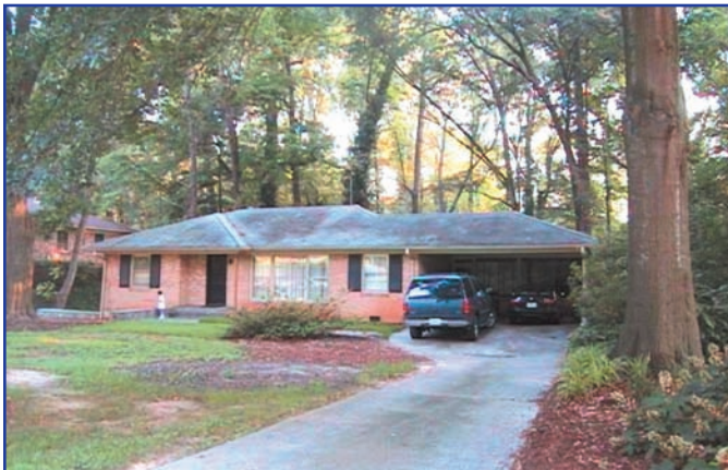
The Cartledge residence in Atlanta, GA was a classic 1950's style ranch. The renovation increased the size of the house to 4,921 sq. ft. from 3,338 sq. ft.
